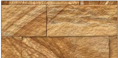
SANDSTONE CLADDING ON PLANTER WALL
