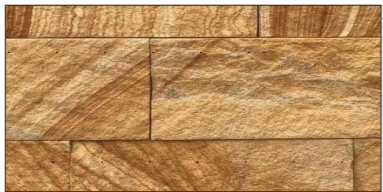
SANDSTONE CLADDING ON PLANTER WALL
